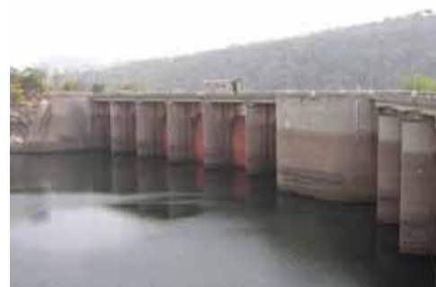
The intake of the Akosombo Dam
