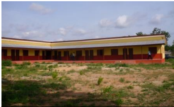
School building for the resettlement communities.
